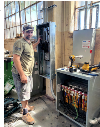
Derek Moeller at work on new Wood Shop electrical panel
