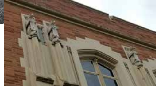
92 years after construction, the North Gym and Auditorium are still faithfully guarded by gargoyles. Photo by Don Cambou
