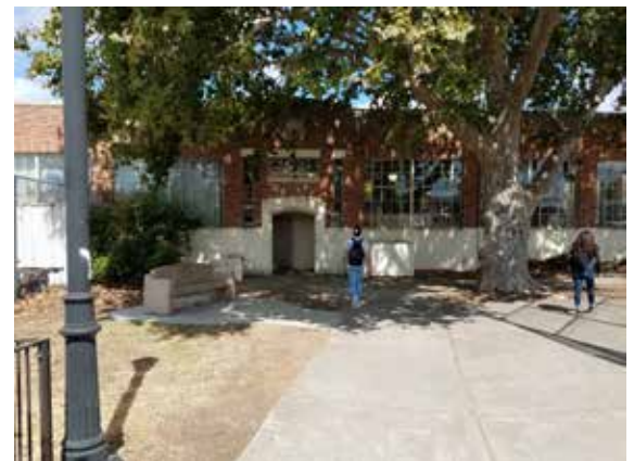
The Wood and Metal shops are now receiving much needed upgrades. Photo Don Cambou
